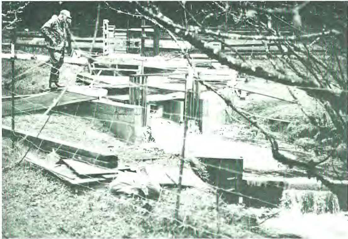
Photo 4. Spillway with concrete steps and adult fish trapping facility at Priorli Creek STEP pond.
